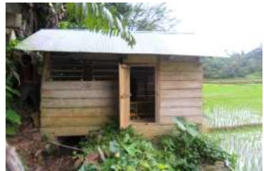
Gambar 10. Gardu sentral (power house) PLTMH Rampusa
